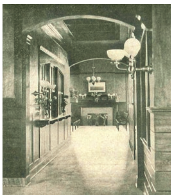
MEMBER DAVID MATTOON FOUND THIS INTERIOR PHOTO OF THE STATION TAKEN SHORTLY AFTER COMPLETION IN 1900 SHOWING THE ORIGINAL WOOD paneled lobby and ticket window, ladies waiting room with fireplace, and gas-electric combination lighting fixtures.
