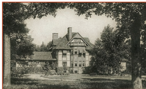
ALICE HOME, LAKE FOREST HOSPITAL'S ORIGINAL STRUCTURE ON THE CAMPUS OF LAKE FOREST COLLEGE.
